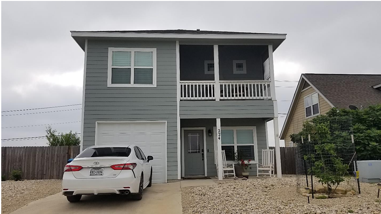
Figure 81: New Single Family Home Construction
